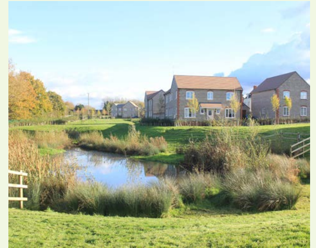
SuDS designed as a natural pond with accessible, split level banks, Ridgeway Farm, Purton Parish, Wiltshire
