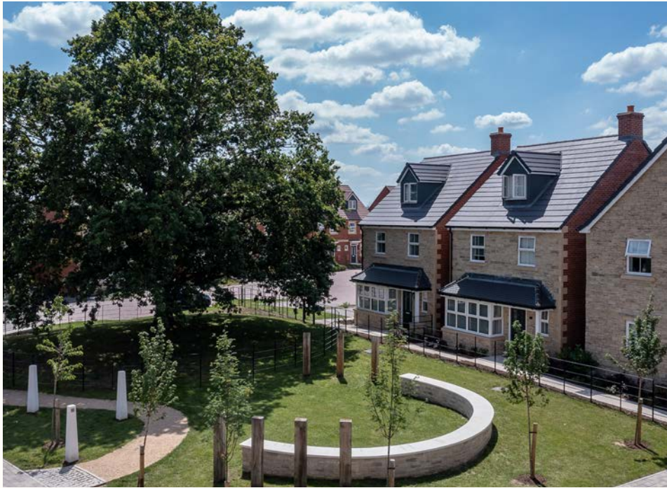
Newland Place, Trowbridge
