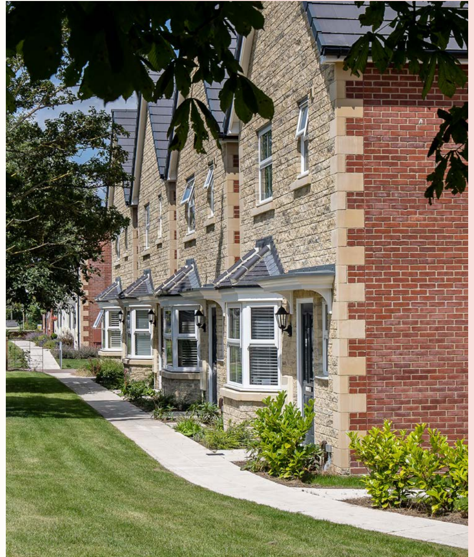
Newland Place, Trowbridge
