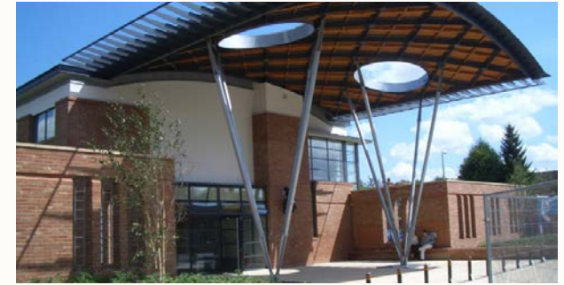
Wiltshire Police Station, Trowbridge
