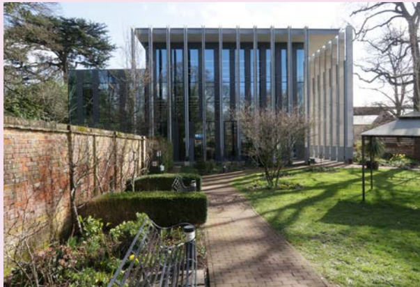
Bourne Hill Council Offices, Salisbury
